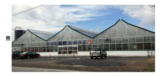
The three-spanned Nexus glass greenhouse has vented roofs, large gables for signage and an expansive automatic sliding door—big improvements over the four hoop houses previously on this site.
