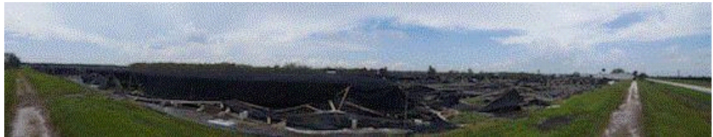
A panoramic view of Heart of Florida shade houses. The complete flattening on the right is indicative of tornado damage.
